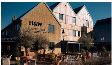
The structure of the building combines a steel frame with a mixture of masonry and timber frame along with beam and block flooring at ground floor level, precast hollowcore planks at first floor level and timber posi-joists at second floor level.
